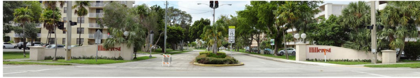
Hillcrest Drive - Existing Conditions
