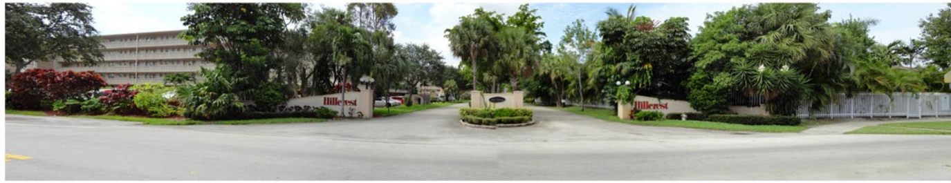
48th Avenue - Existing Conditions
