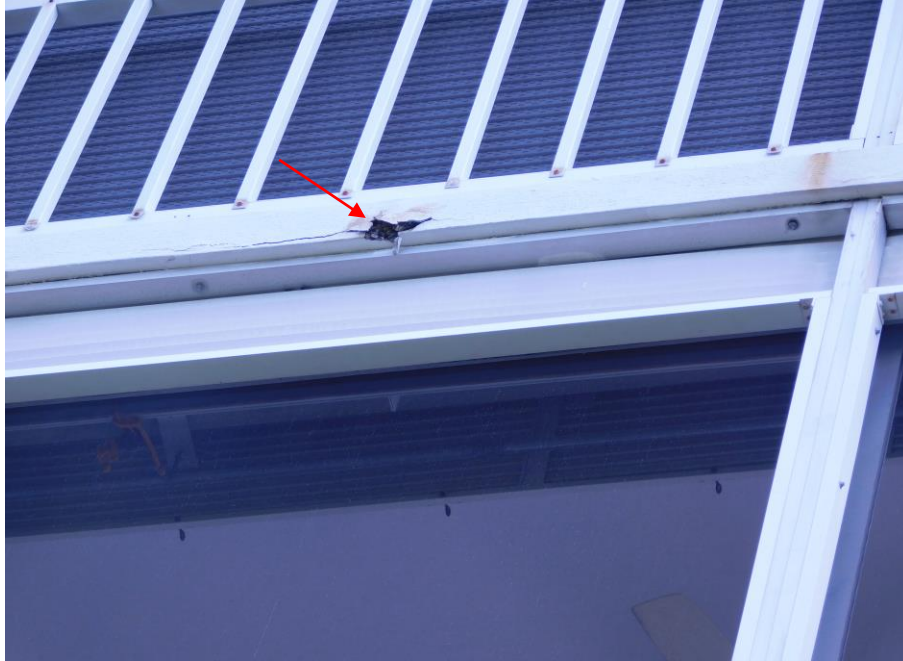
Photo 9: Concrete spalling and cracks on the slab edge.
